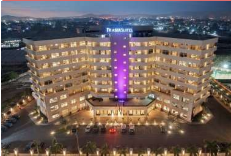
Figure 9: Fraser Suites Abuja: continuous curtain wall with only shallow projecting floor-slab edges
