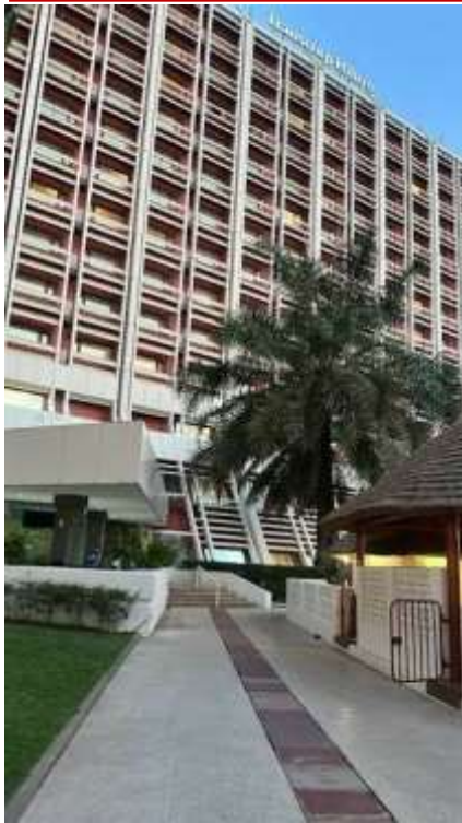
Figure 7: Transcorp Hilton Abuja: massed H-shaped configuration with deep structural balconies
